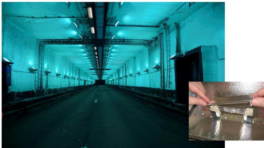
Fig. 5. Final installation of the UV lighting in the Leopold II tunnel during the second main campaign (January 2013). Inset: metallic shutters used to solve the problem of glass heating and subsequent breaking.
