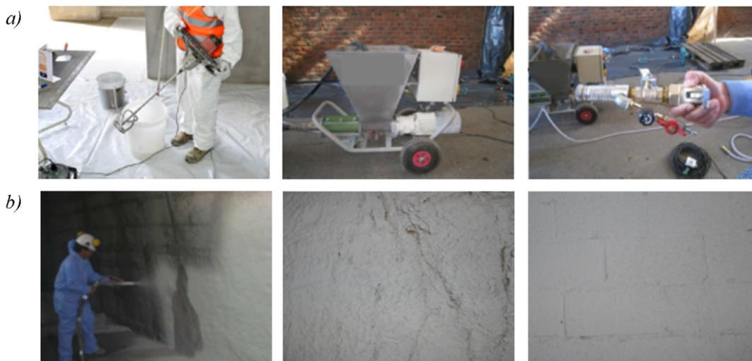
Fig. 4. a) Typical equipment needed for the preparation and application of the photocatalytic cementitious coating material used in the Leopold II tunnel, and b) spraying and associated surface finish on shotcrete and concrete blocks, respectively.
